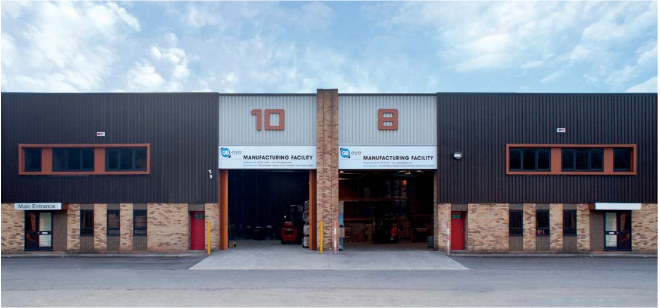
Our framing unit located 1 mile from GB eye's headquarters and Distribution Centre.
